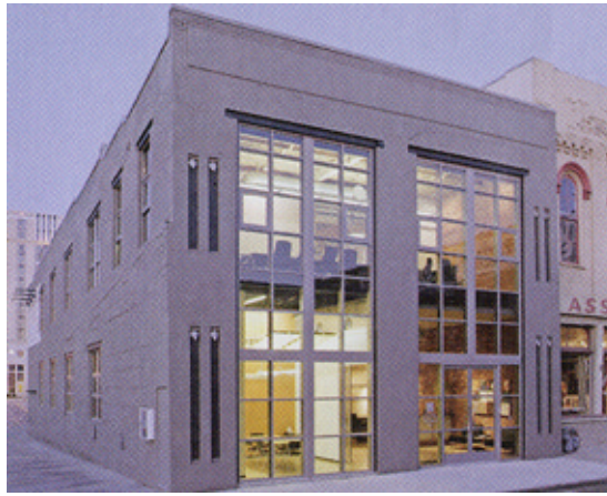
Hastings Architecture Building— Before and after renovation. Large windows were cut in and added at the originally solid brick southern face of the building in conjunction with the use of interior glass.
