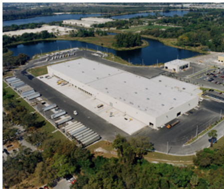
FedEx AGT&T/DGO Facility, Hollywood, FL
